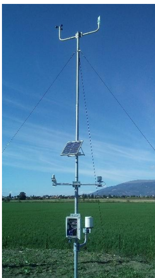
PF5-55 - Pole h=5m with guy wires
